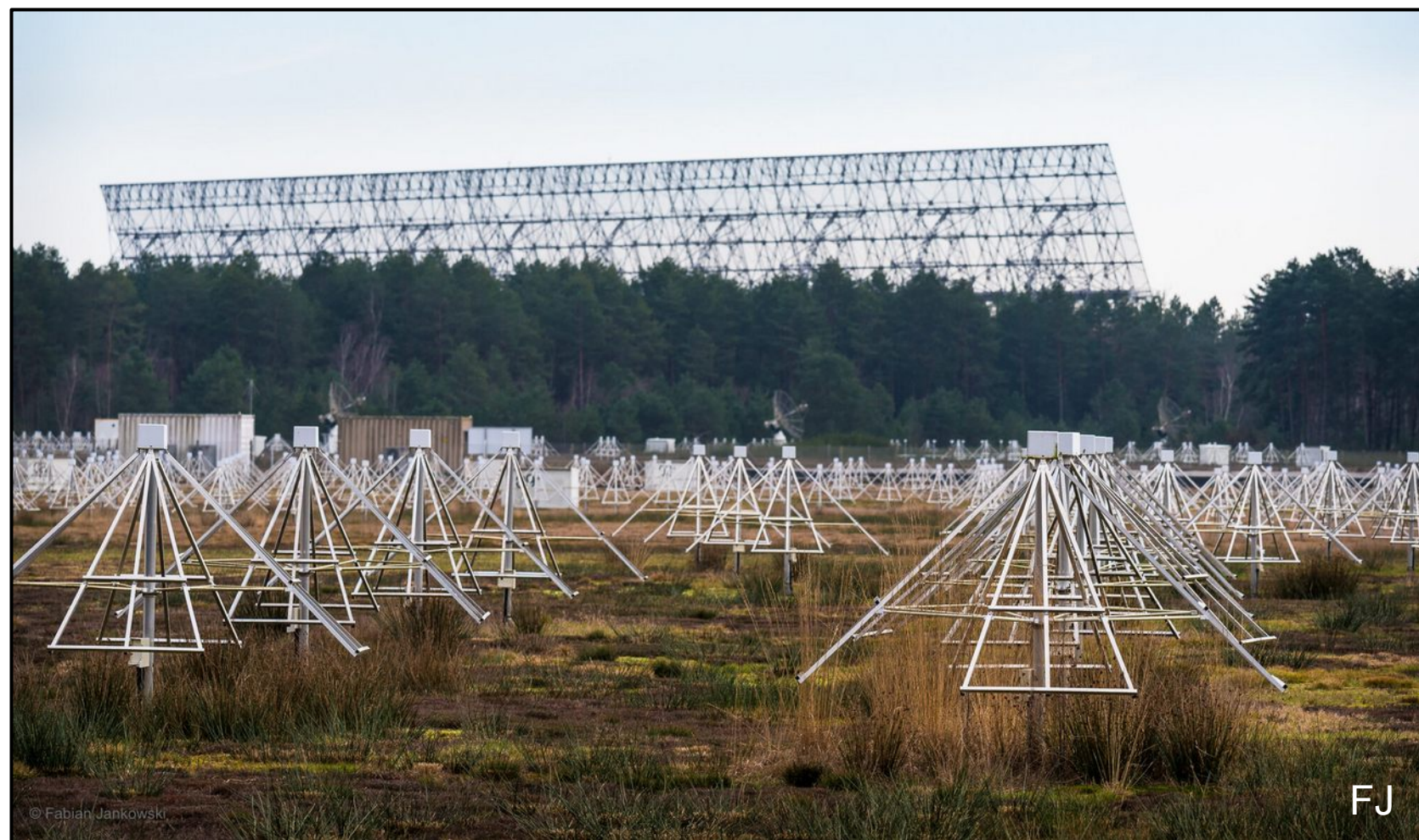
Fig. 1: The NenuFAR telescope (10–85 MHz) in front of the LOFAR FR606 HBA antennas (110–240 MHz) with the NRT (1.1–3.5 GHz) in the background.
